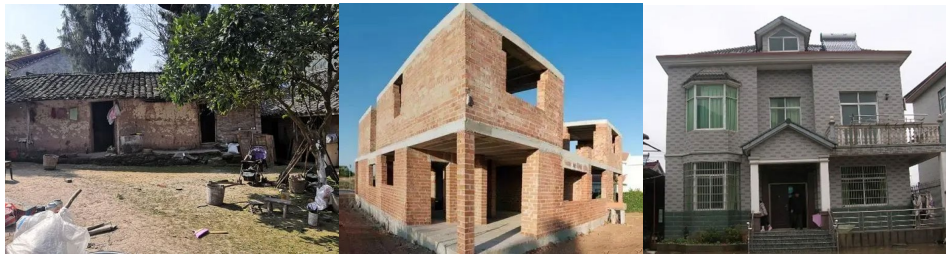
Fig. 3. Common forms of rural houses in Xuzhou.
