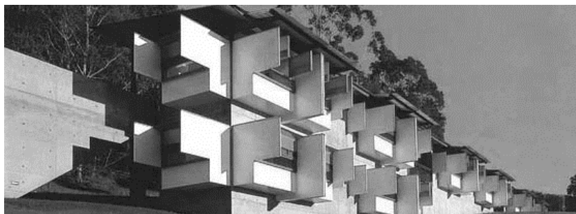
Fig. 5. Application of facade shading.
