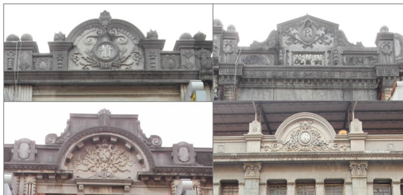
Fig. 3. Gable of the houses in the Qishan old street.
