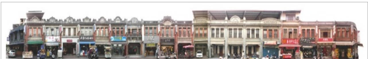
Fig. 2. Facades of houses in the Qishan old street.
